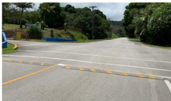
FEBRUARY 25 & 26 SPEED BUMP STRIPES Our maintenance staff revamped the speed bumps by repainting the stripes for visibility to help ensure safety for our pedestrians and drivers.
